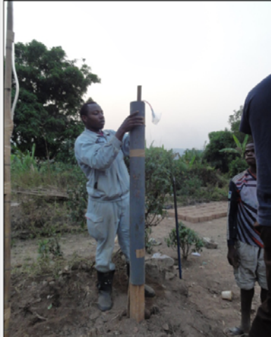
Fig. 3 Installation of rainwater collector
