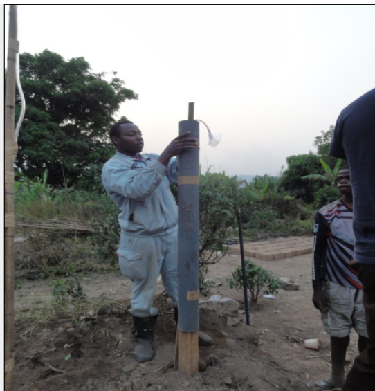
Fig. 3. Installation of rainwater collector
